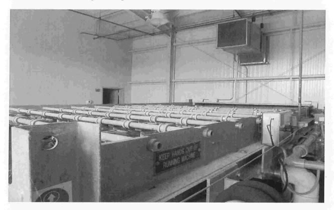
Photo 16 – Gravity belt thickener for sludge
