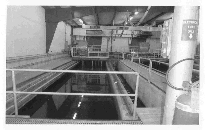
Photo 18 – One of the traveling bridge sand filters
