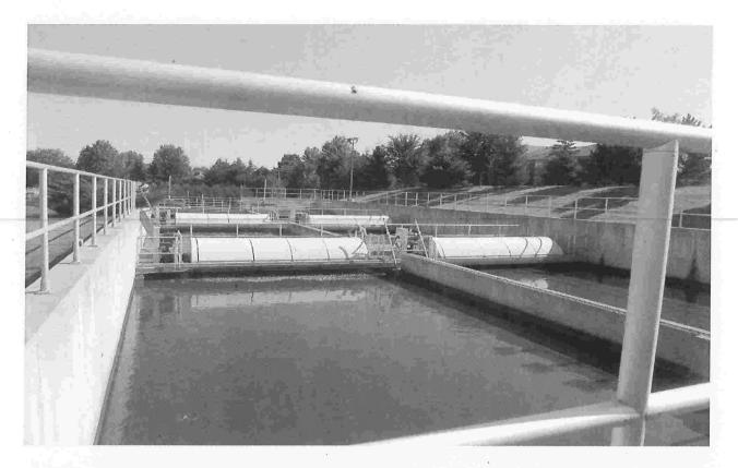
Photo 5 – Vertical loop reactor (VLR)
