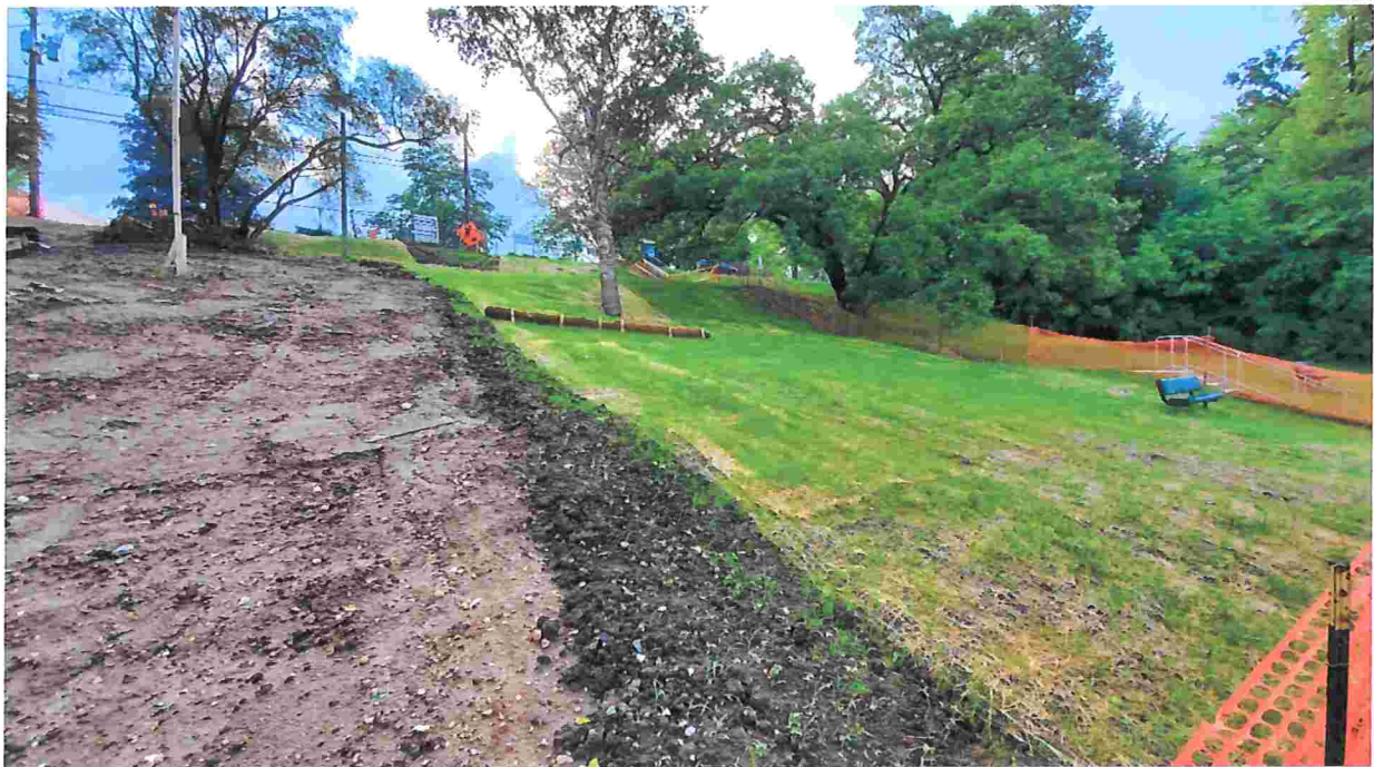
Hagele Beach Hill Restoration
