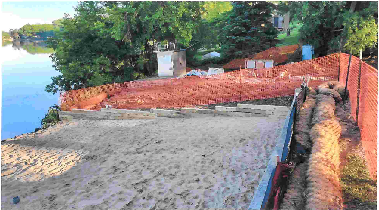
New Beach Retaining Wall
