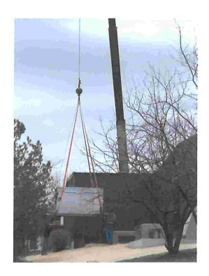
Delivery and placement of new Make-Up Air Units for the Filter Building
