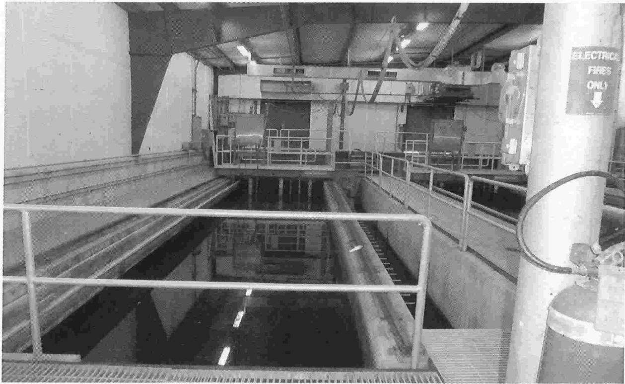
Photo 18 – One of the traveling bridge sand filters
