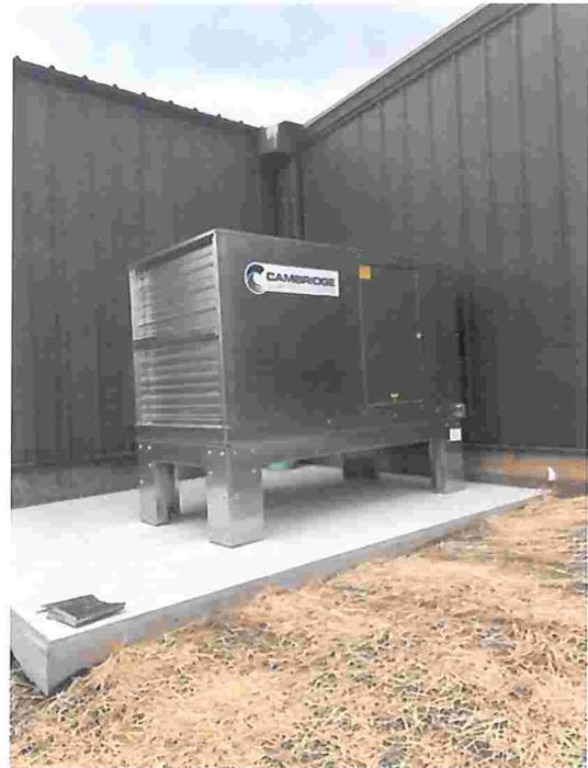
Exterior and interior installation of Make-Up Air Units, including temporary platform.
